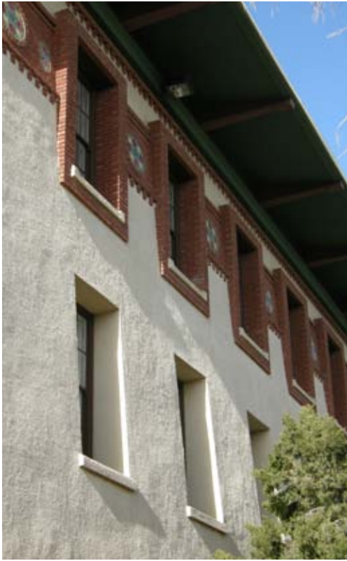
Stuccoed masonry wall at Old Main
