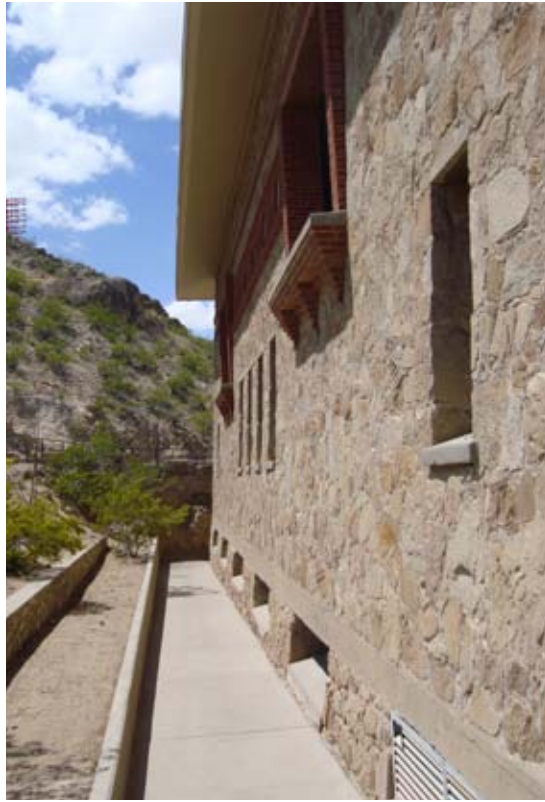
Uncoursed stone wall at Holiday Hall
