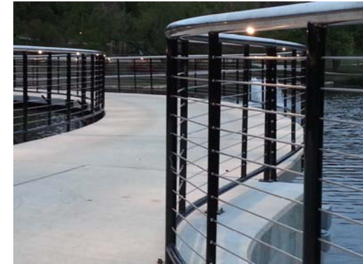
Handrail Puck Lights
